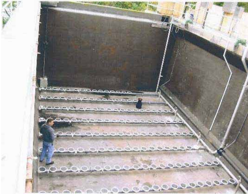
NEWLY INSTALLED FINE BUBBLE DIFFUSERS Photo Courtesy of Northport WWTP
