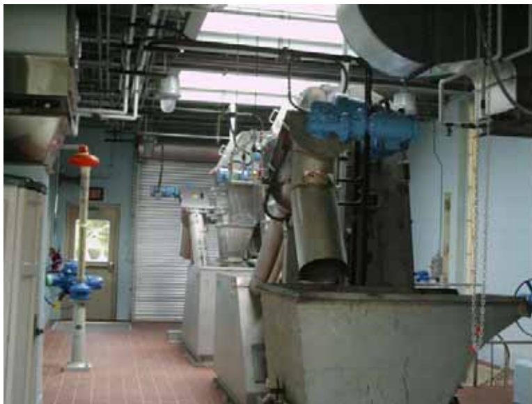
FINE SCREENS AND SCREENING INSIDE RENOVATED AND EXPANDED BUILDING Photo Courtesy of TOMSA
