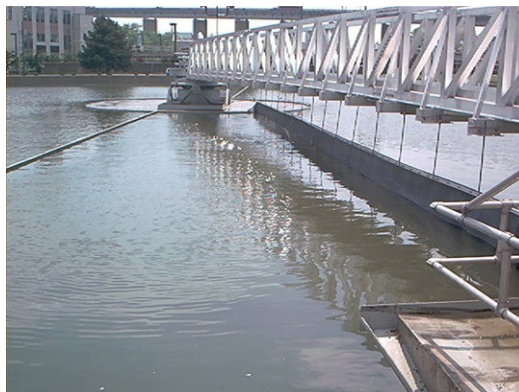
NEW BRIDGE AND SCUM BAFFLE Photo courtesy of Joint Meeting
