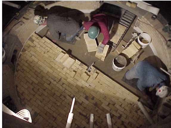
INTERIOR BRICKWORK IN NEW INCINERATOR Photo courtesy of West Haven WPCC
