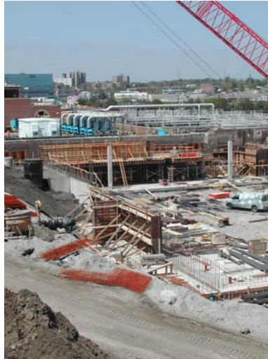
AERATION TANK UNDER CONSTRUCTION Photo courtesy of Stamford WPCA
