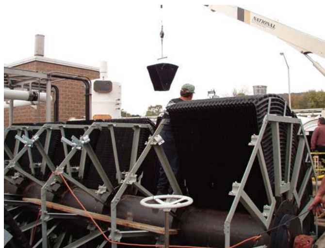
ROTATING BIOLOGICAL CONTACTOR INSTALLATION
