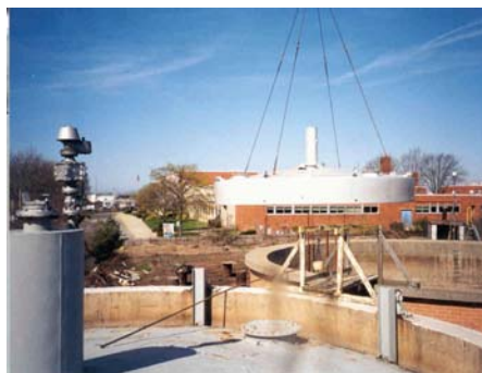
DIGESTER COVER INSTALLATION
