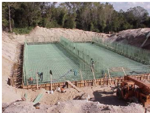
NEW SEQUENCING BATCH REACTOR TANKS
