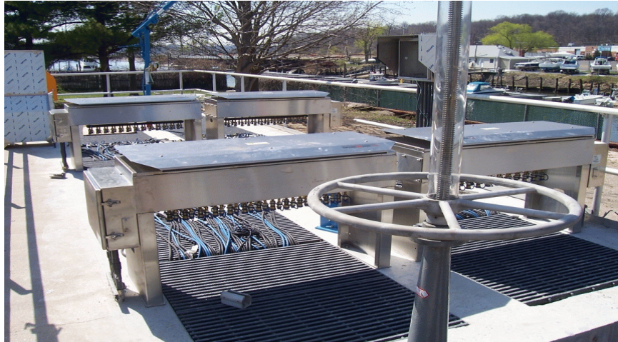
NEWLY INSTALLED UV DISINFECTION Photo Courtesy of Cameron Engineering
