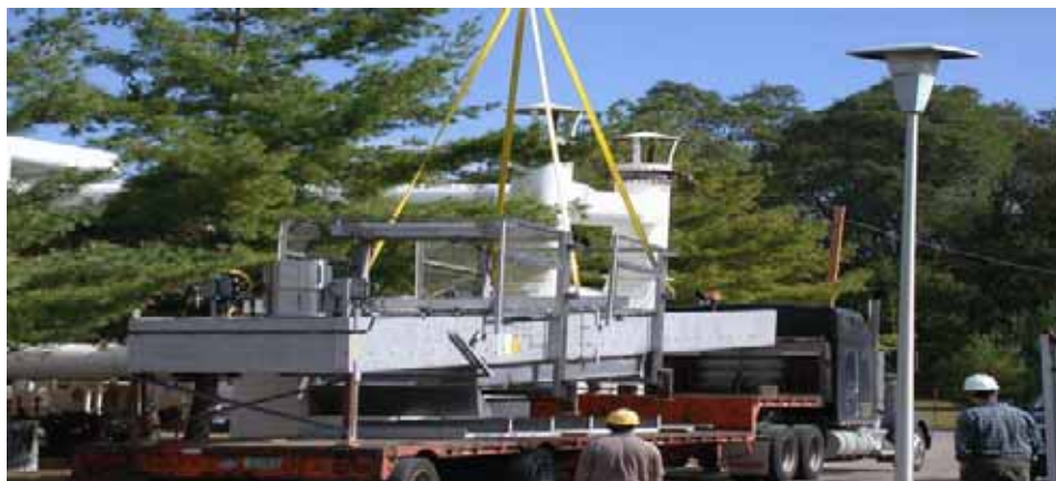
BAR SCREENS BEING OFF-LOADED
