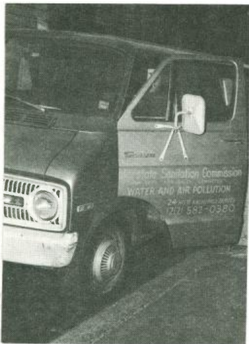
Mobile Air Sampling Unit. Van is used for on-site measurement of air pollutants and for special studies, such as the benzene sampling program.
