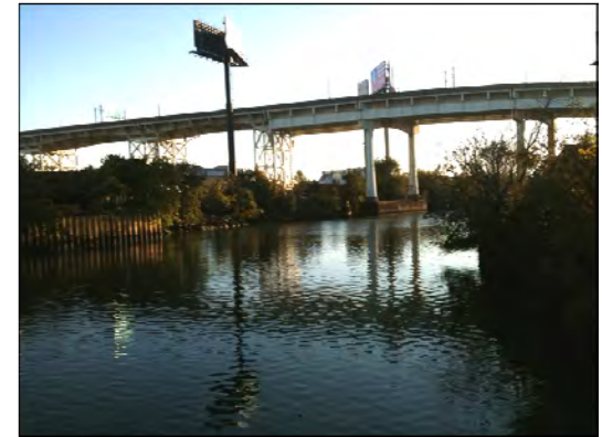
The Long Island Expressway over Dutch Kills
