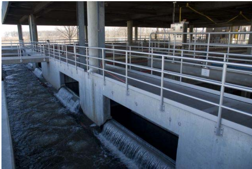
Effluent wastewater leaving the sand filtering process
