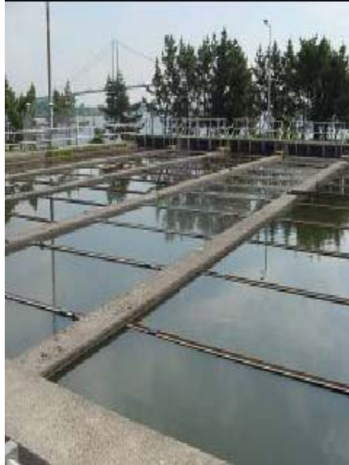
New Settling Tanks Photo Courtesy of NYC DEP
