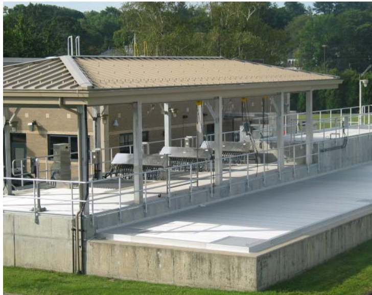
New UV System Photo Courtesy of Grass Island WWTP
