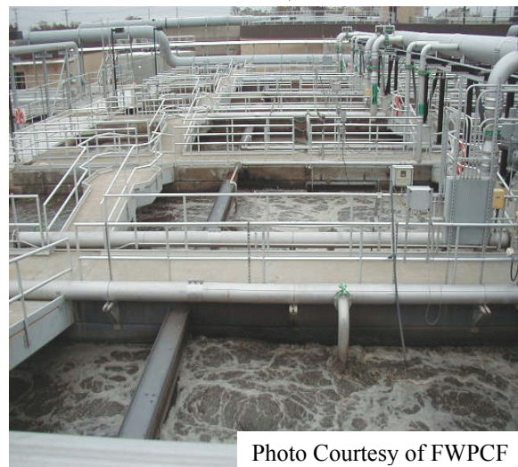
EXPANDED DENITRIFICATION TANKS
