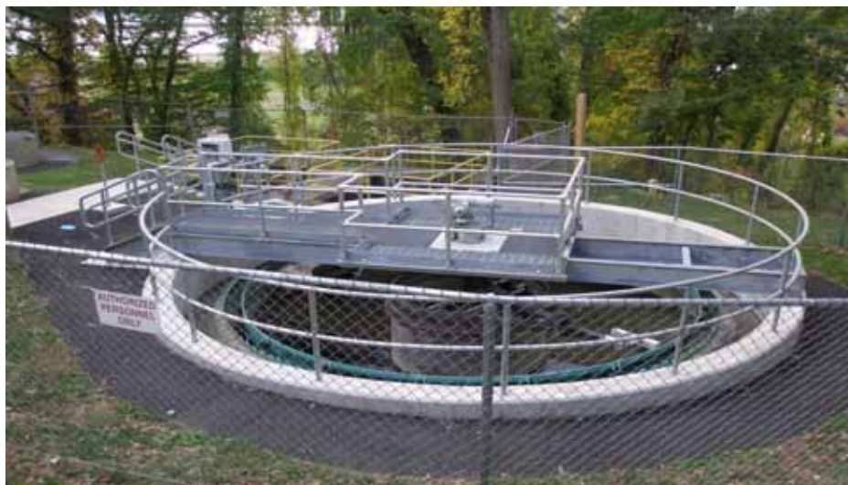
New Final Clarifier Photo Courtesy of R. Morlock, WWTP Supervisor, Camp Smith
