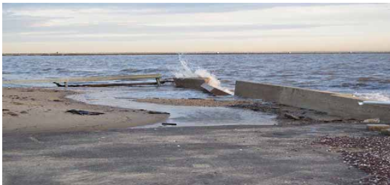
Destroyed Seawall at Leonardo, New Jersey, March 2010
