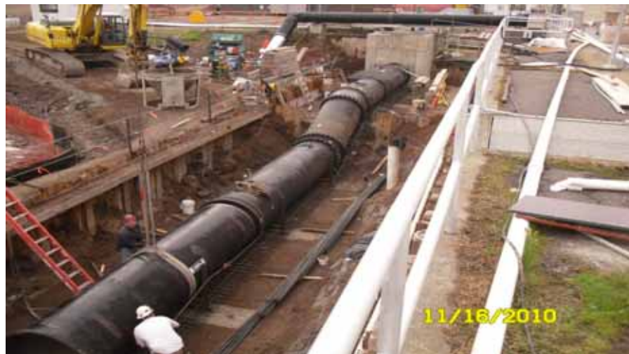
New 48-inch Effluent Line from Secondary Clarifiers to Chlorine Contact Tank Photo Courtesy of West Haven WPCP
