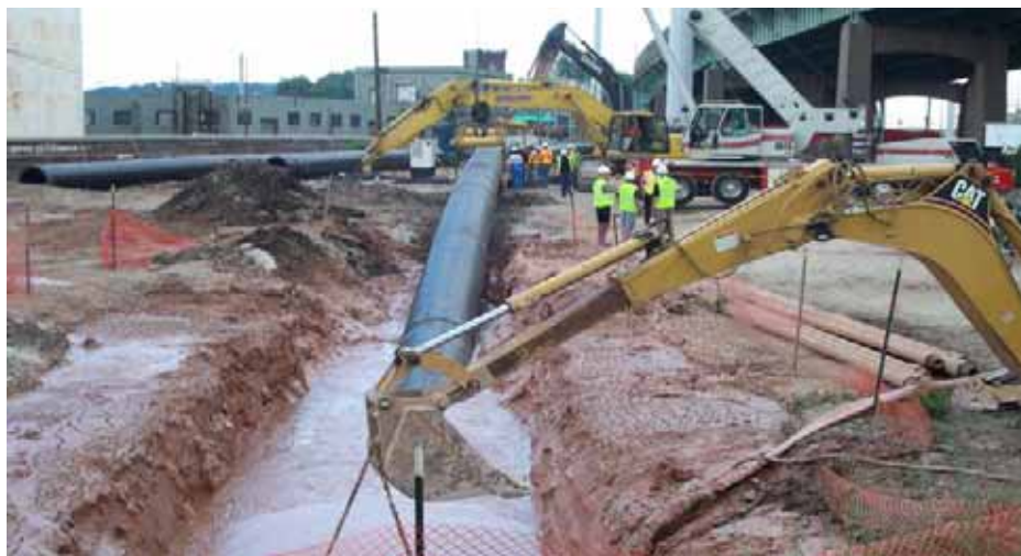
Twin 42-inch Force Mains Being Installed Beneath New Haven Harbor Photo Courtesy of GNHWPCA
