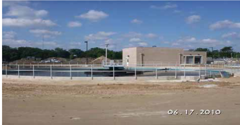
New Final Clarifier, and Return Sludge and Blower Buildings Photo Courtesy of TOMSA
