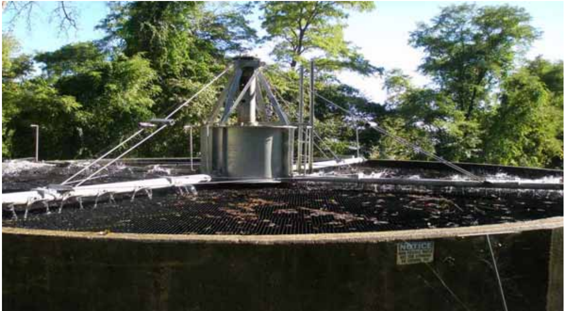
Refurbished Trickling Filter with New Distribution System and Media Photo Courtesy of R. Morlock, WWTP Supervisor, Camp Smith
