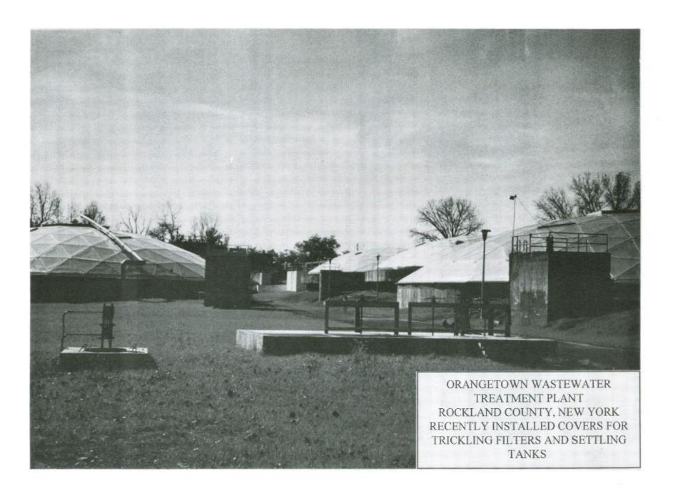
an SSES (completed 1993), to institute a short-term plan to improve the existing trickling filters, and to upgrade and expand the plant capacity to 12.75 MGD. Construction was completed in October 1996. Final costs were estimated at \$8 million for all construction phases including a primary clarifier, a trickling filter, and a secondary clarifier, as well as refurbishing miscellaneous mechanical equipment.
