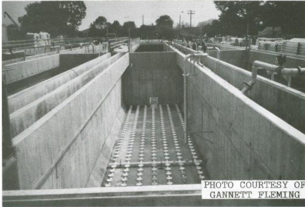
FINAL AERATOR WITH FINE BUBBLE DIFFUSERS
