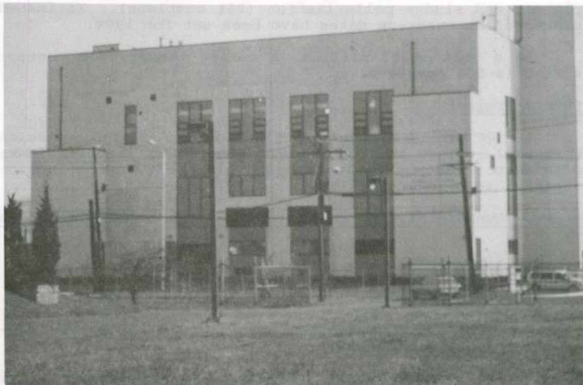
SLUDGE HANDLING FACILITIES
