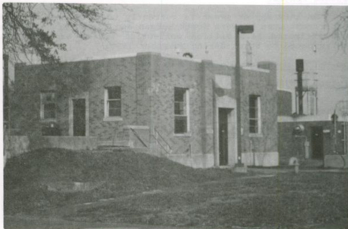
SODIUM HYPOCHLORITE BUILDING
