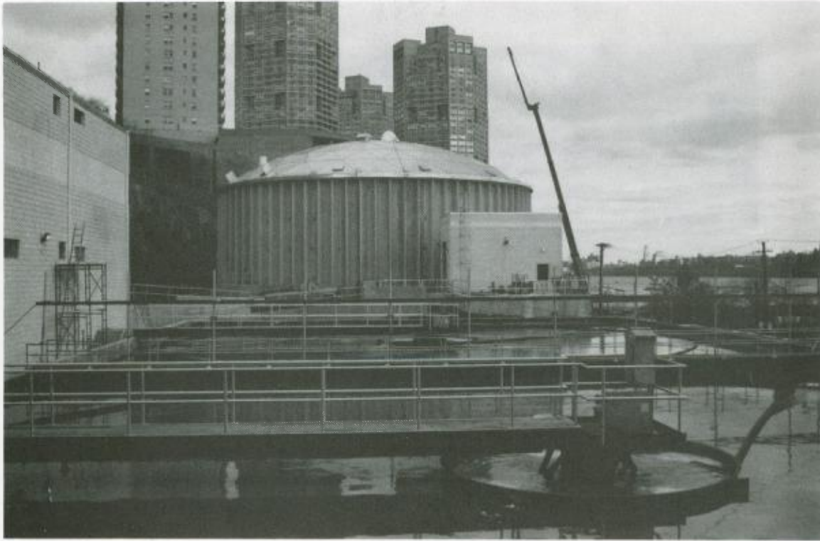
Refurbished Settling Tanks
