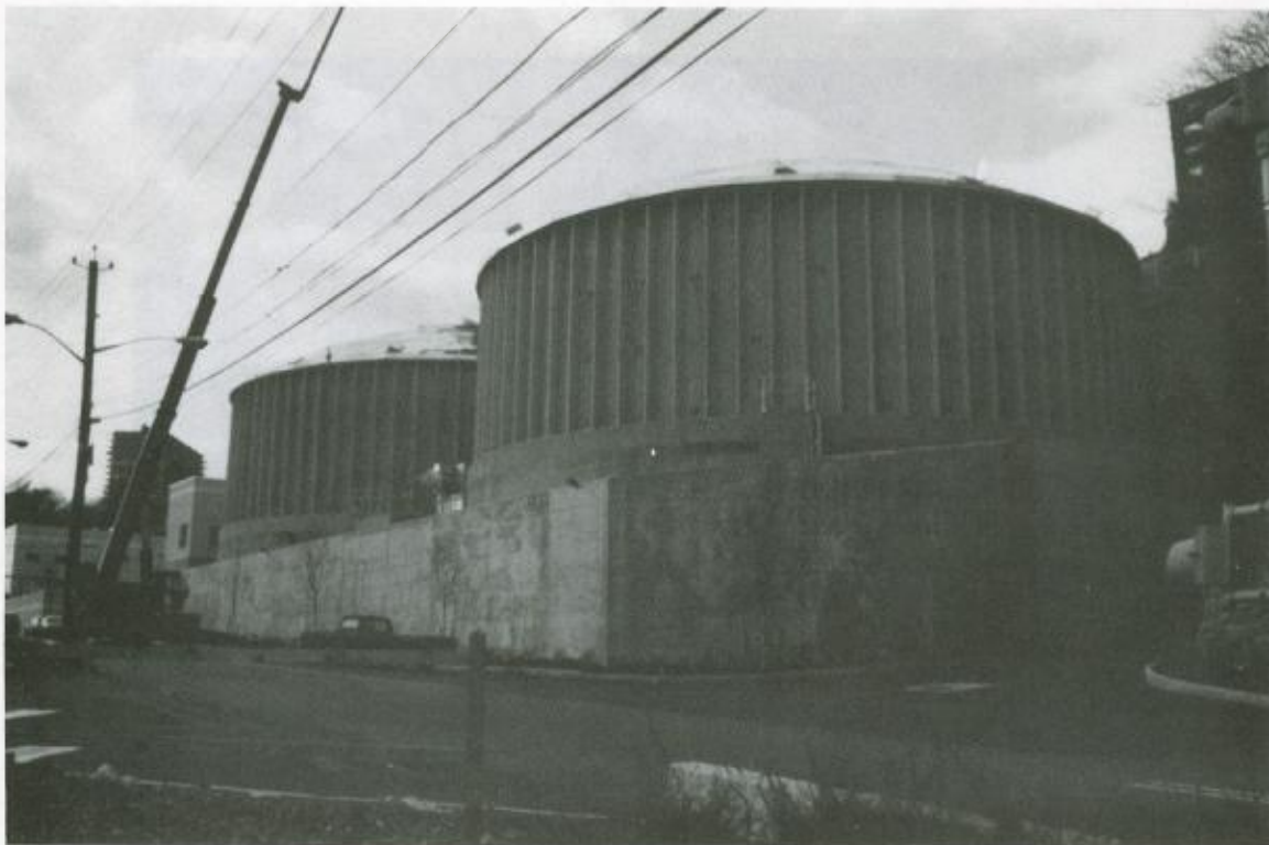
Enclosed Trickling Filters
