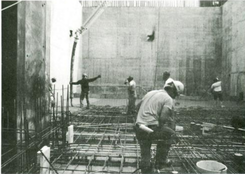
WOODBRIDGE AVENUE PUMP STATION CONSTRUCTION
