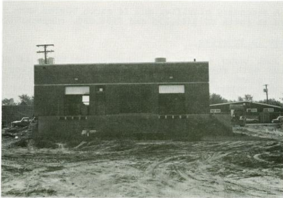
Pump Station Building
