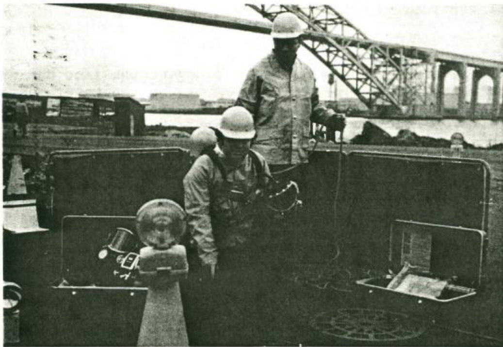
FIG. 9-A, STANDARD PREPARATION AND SET-UP FOR REGULATOR INSPECTION
