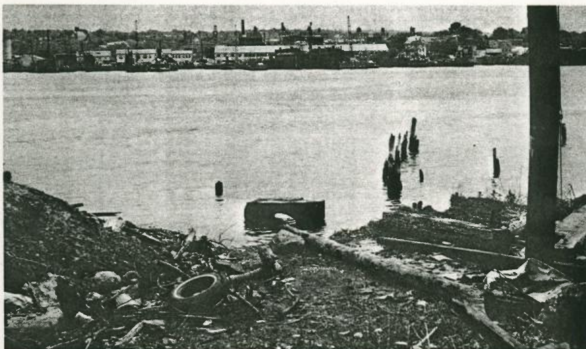
FIG. 50-B, OUTFALL FOR REGULATOR 5, INGHAM AVENUE AND EAST 5TH STREET, BAYONNE, NEW JERSEY
