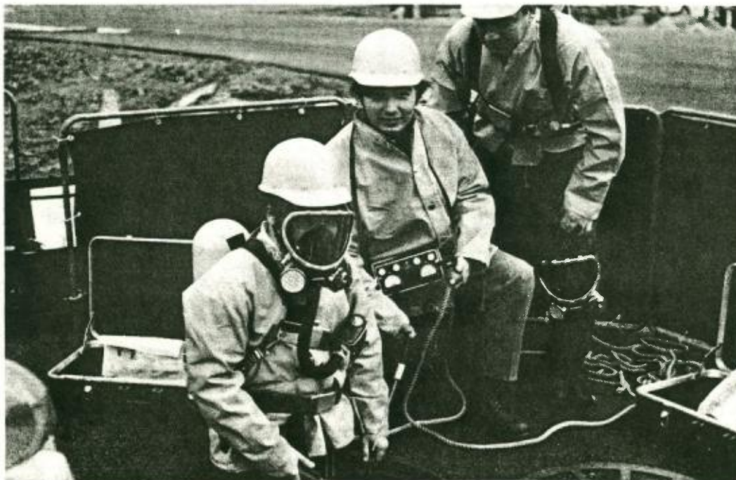
FIG. 9-B, FIELD PERSONNEL ENTERING MANHOLE FOR REGULATOR INSPECTION
