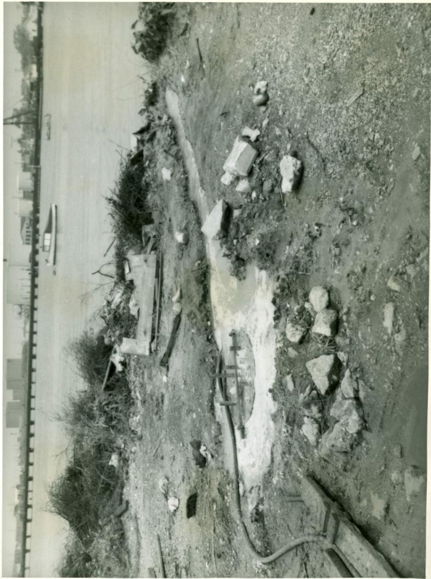
FIG. 1. Overflowing manhole at Riverside Blvd. and Water Street. Hose at left is used for applying chlorine Reynolds Channel in background.
