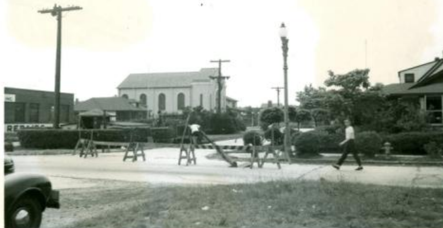
Fig.4 West Park Ave. and Lindell Blvd. Temporary pumping operations to relieve surcharged sewer.
